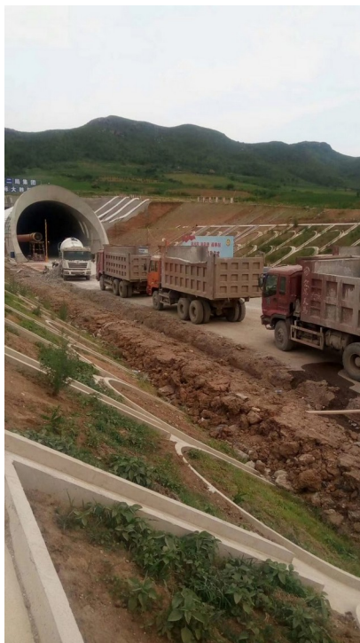
A tunnel portal, with dump trucks and a cement mixer lined up to go in. Photo by Yanlin Zhao.
